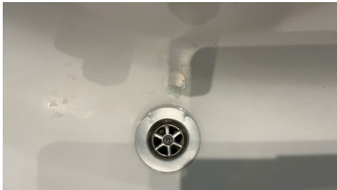
Riss i vask
