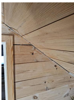
Overflate vegg - Gliper mellom panelbord.
