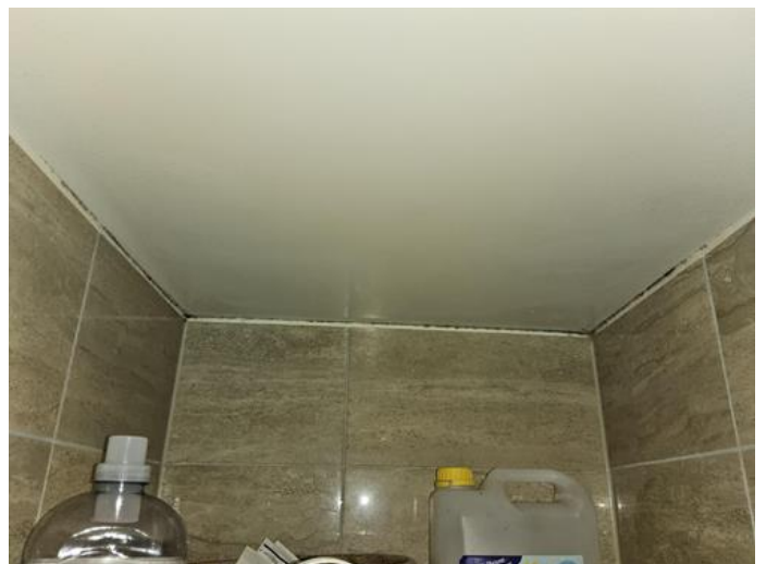
Overflater himling - [Svertesopp over vaskemaskin ]
