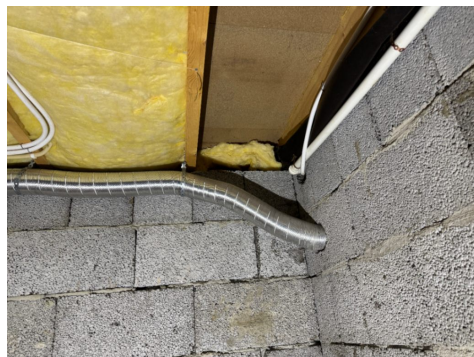
Manglende isolering
