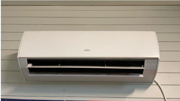
Varmepumpe - innerdel.
