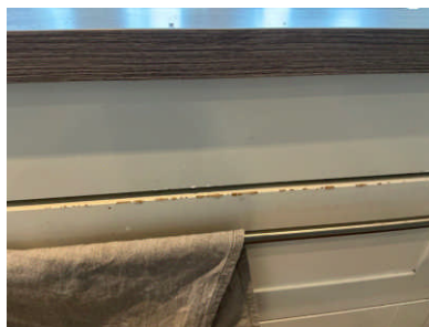
Skader i front under vask.
