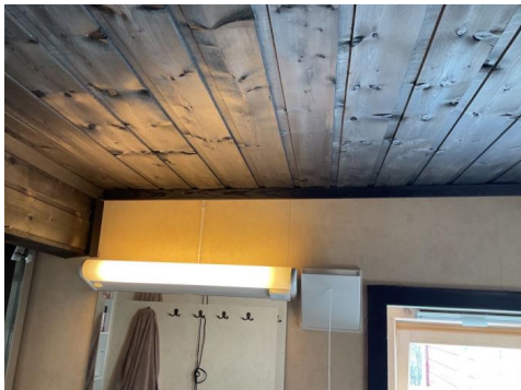
Trepanel i taket.
