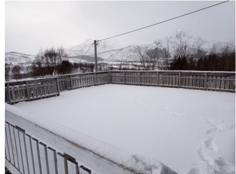
Veranda over carport
