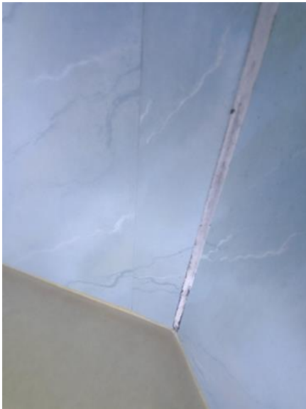
Overflater vegger - [IMG_20250310_113931]
