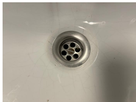
Riss/krakelering i servant.
