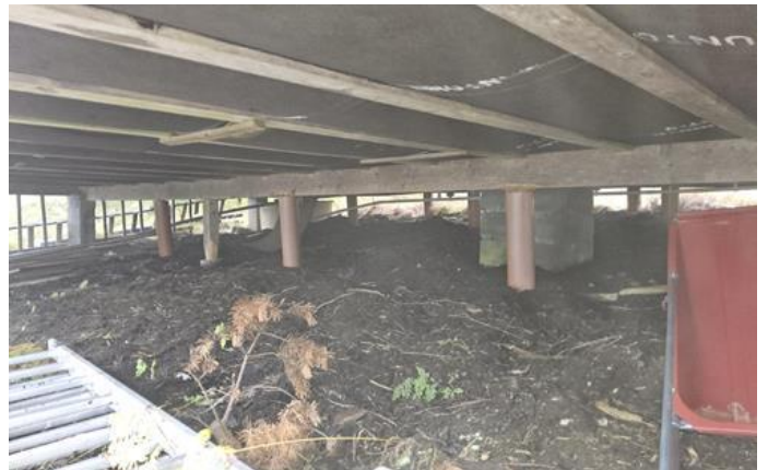
Grunnmur, fundamenter - [IMG_20241017_104240]
