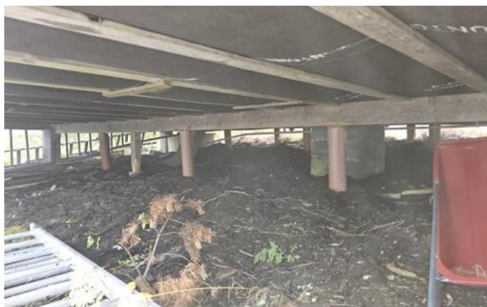
Grunnmur, fundamenter - [IMG_20241017_104240]
