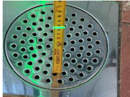
Fallforhold - ca. 125 mm topp slukrist
