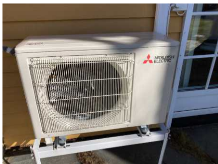
Varmepumpens utedel.
