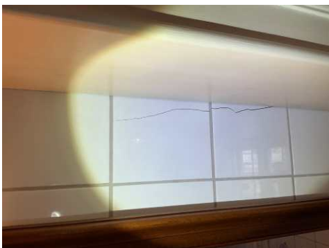
Horisontal sprekk over speil
