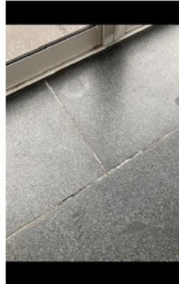
Balkonger, terrasser, veranda etc - [Flisfuger innglasset veranda]
