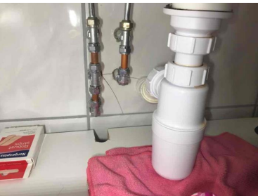
Sprekker i flis under servant.
